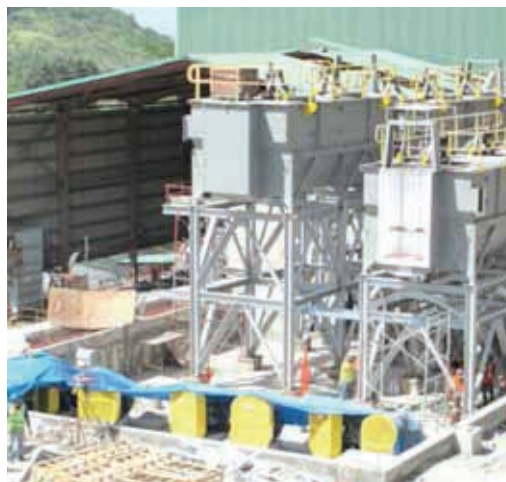
NOV 2013: Installation of high-grade cleaners
