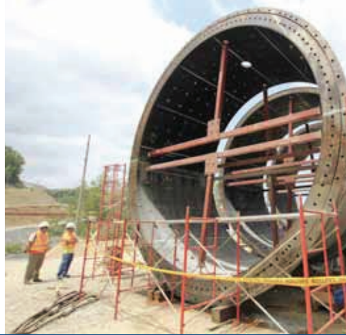
FEB 2013: Assembling of ball mill parts at laydown area no. 1
