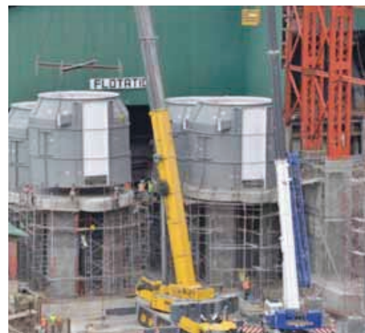
SEP 2013: Installation of TC300 Rougher Flotation Cells
