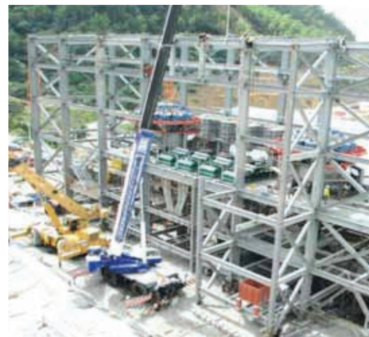
DEC 2013: Installation of cyclones
