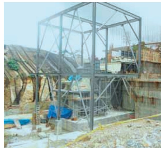
JUN 2013: Installation of jaw crusher
