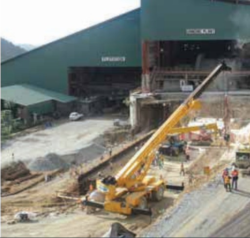
JAN 2013: Groundworks and civil engineering works
