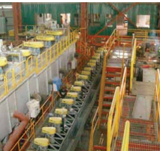
OCT 2013: Construction at the molybdenum plant project
