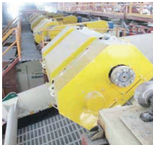
MAY 2013: Installation of vibrating banana screens
