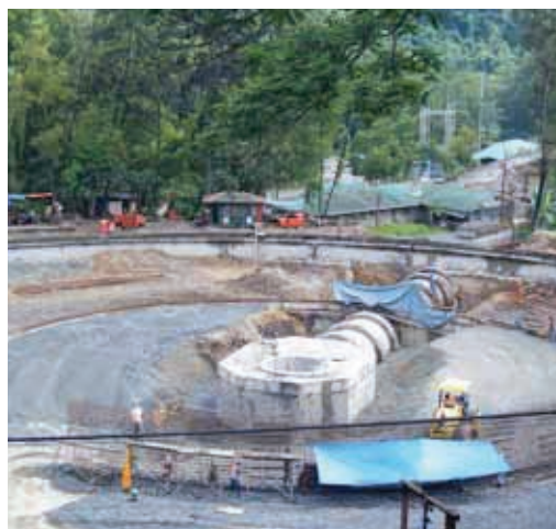
AUG 2013: Upgrading of tailings thickeners
