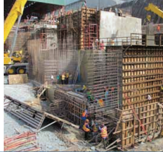
MAR 2013: Construction at the ball mill area
