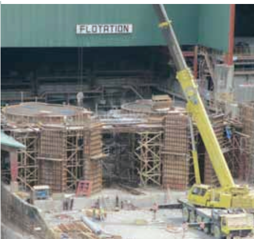
JUL 2013: Civil works at the new TC300 flotation cells area
