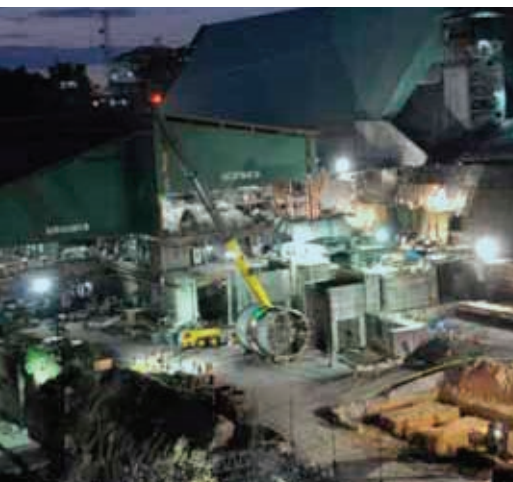
APR 2013: Installation of Ball Mill #9
