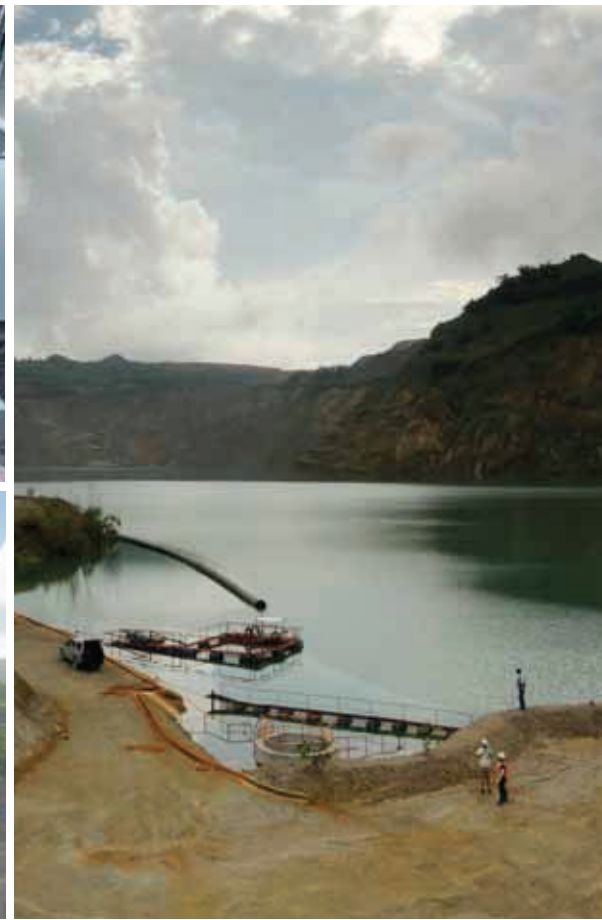
Biga Pit tailings storage facility
