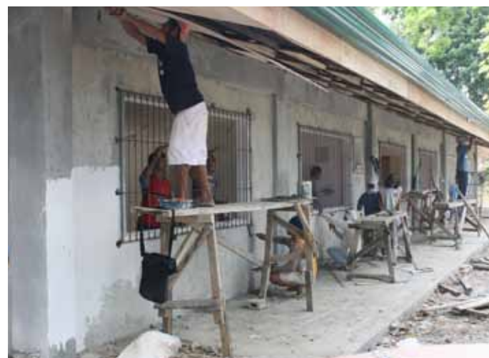
Construction and repair of classrooms
