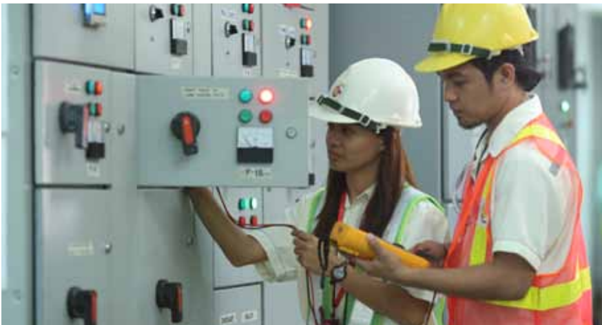
Safety first at the Motor Control Center
