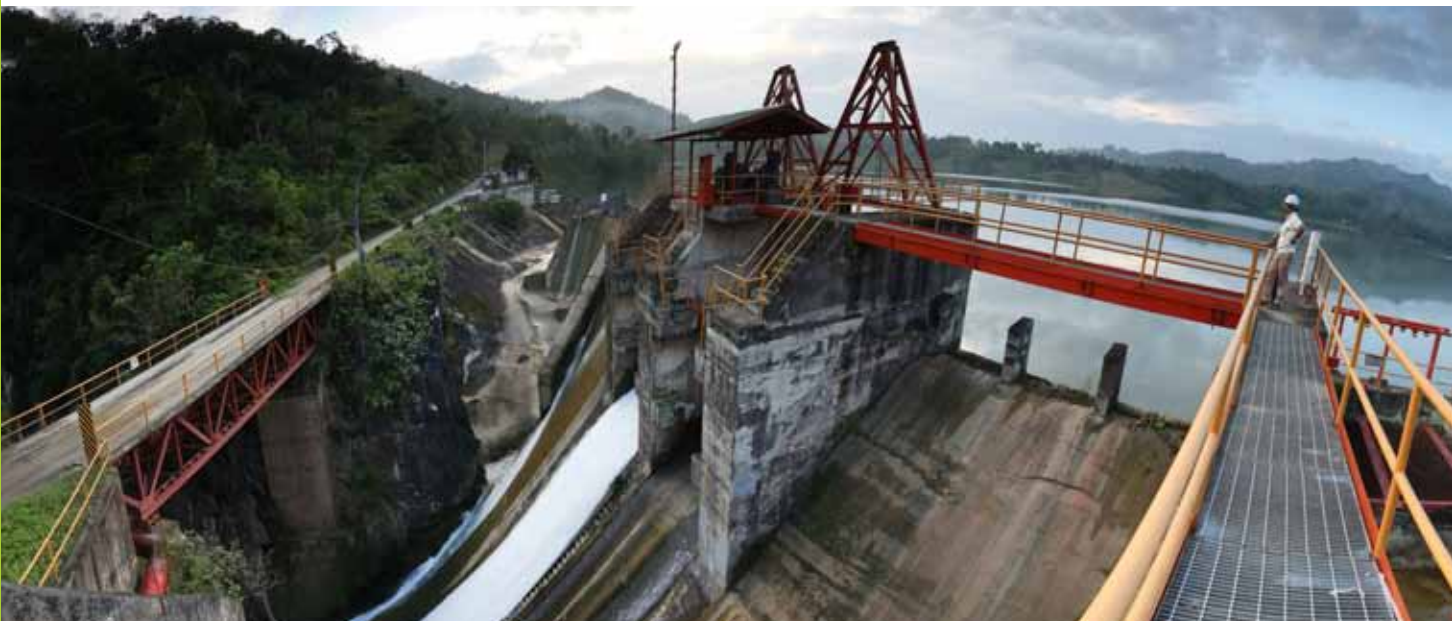
Malubog Dam floodgates
