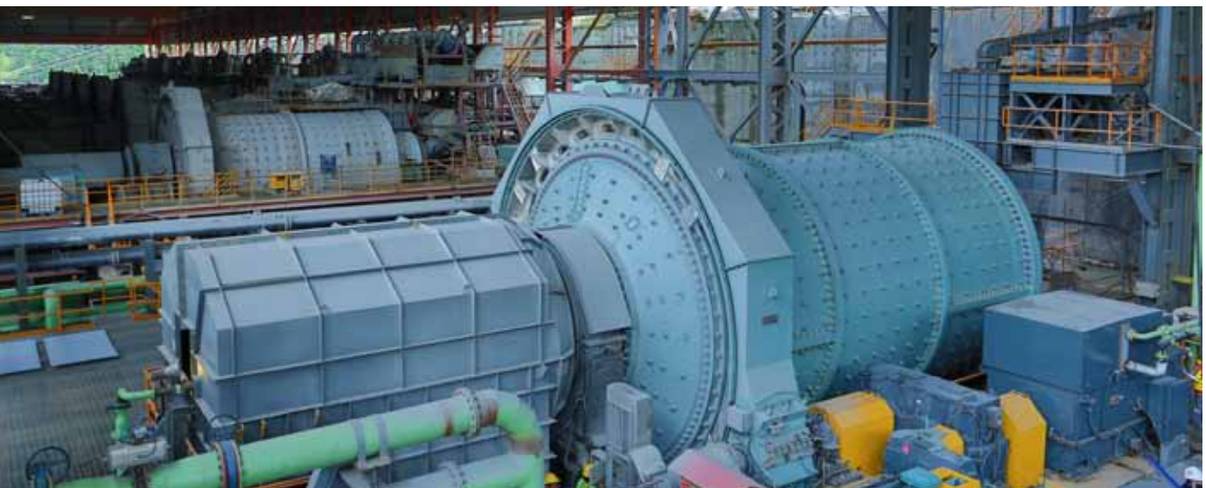
Clockwise from top left: Loading of copper ore, high-grade cleaner, tailing pipelines, ball mills and flotation cells
